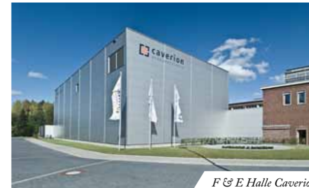
F & E Halle Caverion
