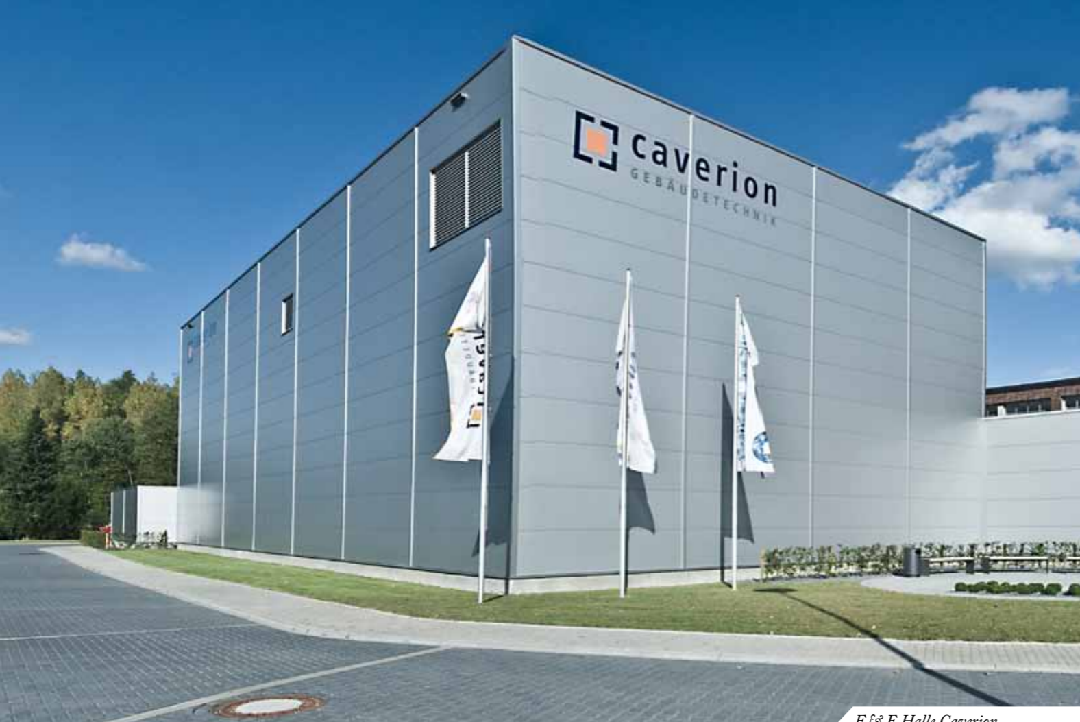
F & E Halle Caverion
